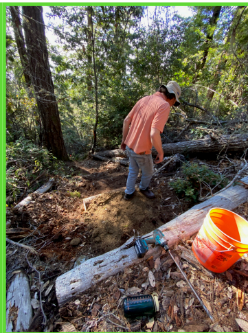
John Howland and logs reinforcing bottom of hillside.
